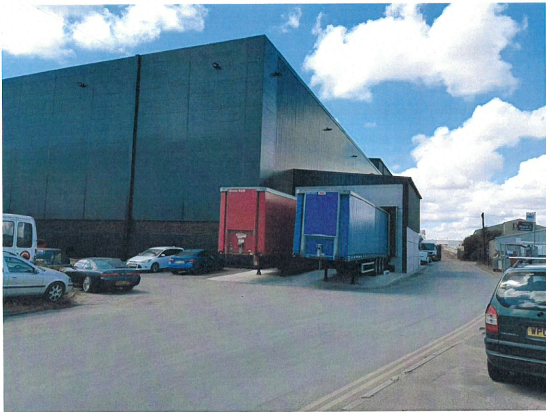
Photograph 1: Existing HGV loading Bay
