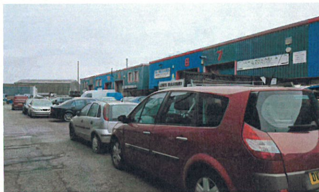
Photograph 6: Existing Conditions on Between Units 1-11 RJMC and Spitfire House
