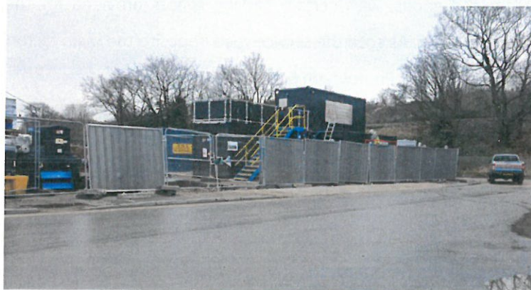
Photograph 3: New Warehouse Construction
